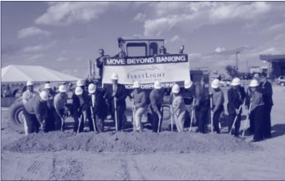
FirstLight Federal Credit Union Executive management, members from the Board of Directors and other key members of the Las Cruces business community joined together to celebrate the groundbreaking of a new branch at 3791 E. Lohman in Las Cruces, NM. Photo provided by FirstLight FCU.
