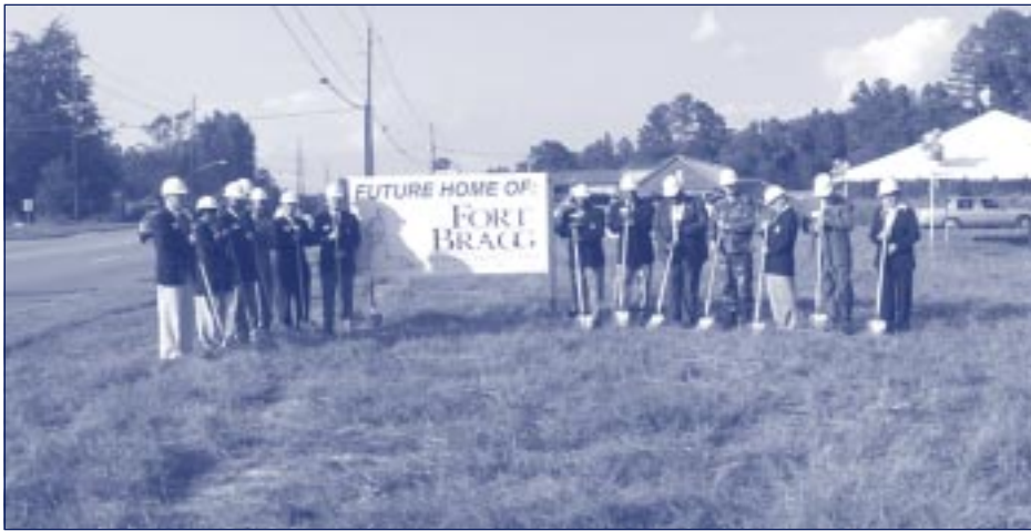
Fort Bragg FCU breaks ground for new Branch. Photo provided by Fort Bragg FCU
